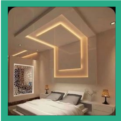
Gypsum False Ceiling
